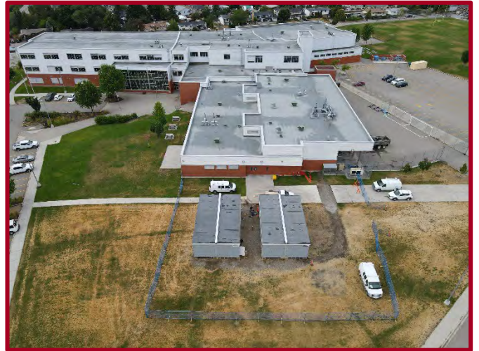
VSS -2 new Modular classrooms
