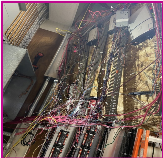
BX DDC upgrade and support office renovation!!
