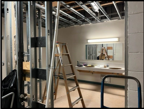
Bathroom Renovations at Kal underway
